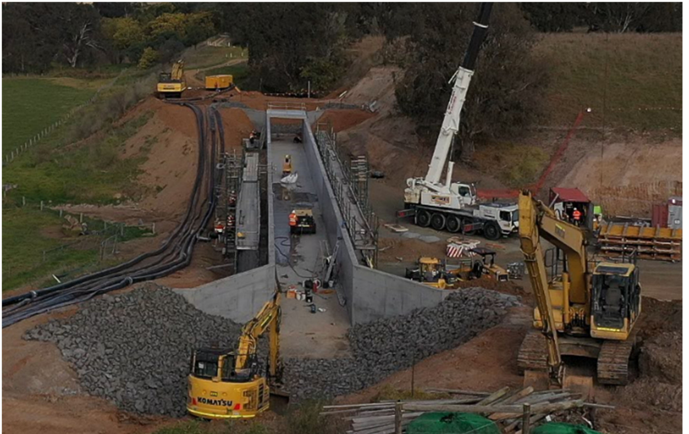
Main Northern syphon to flume.
