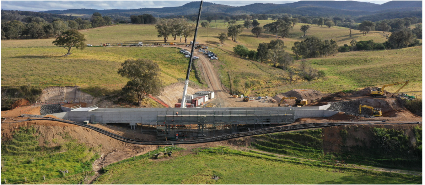
Main Northern syphon to flume
